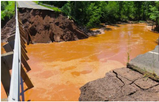
Road washouts like this one occurred throughout the Western U.P. as a result of heavy storms in July 2016.
